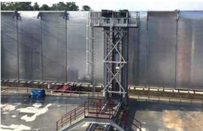
Use of roller shutters in a Single Chamber System
